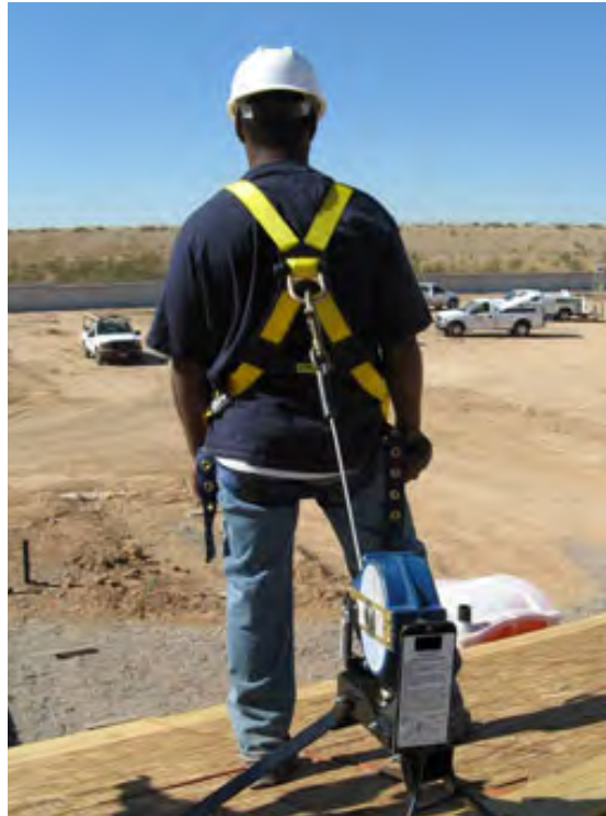
An employee is outfitted with residential fall protection. (Photo from www.OSHA.gov .)
